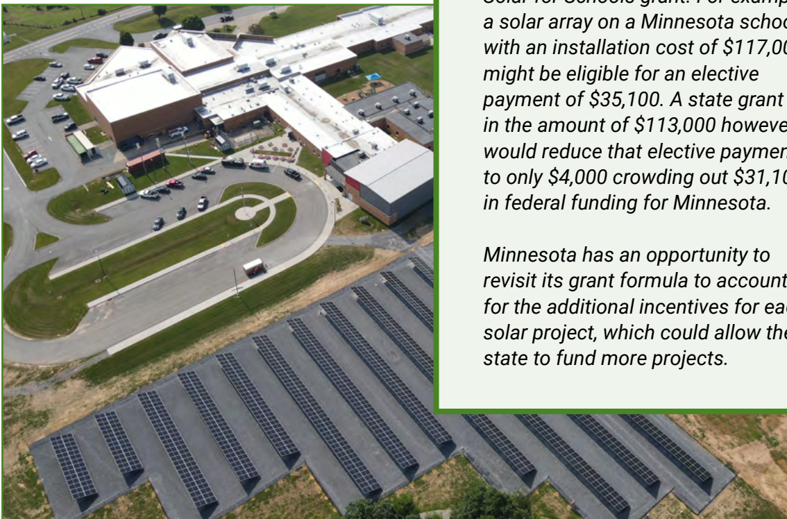
Aerial view, solar panel array at Rupert Elementary and Western Greenbrier Middle. Greenbrier County School District, West Virginia. Courtesy of CMTA.
